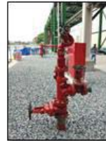
● Fire Hydrant with Monitor
